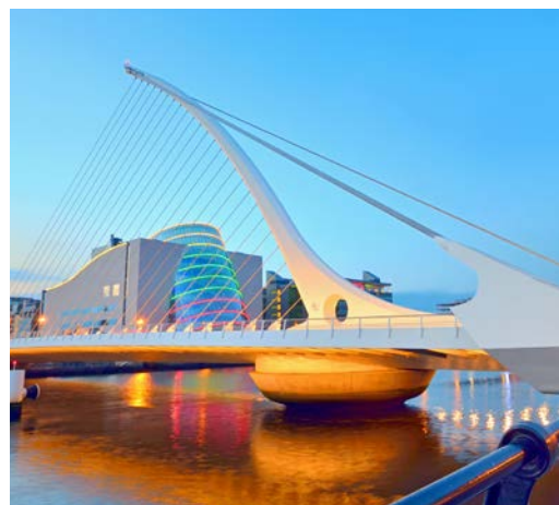
Samuel Beckett Bridge - Dublin Quay
